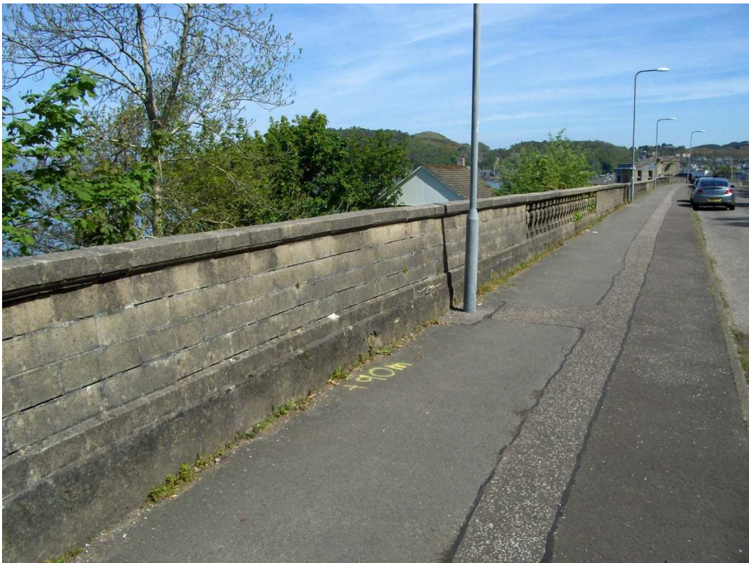
General view of South wall
