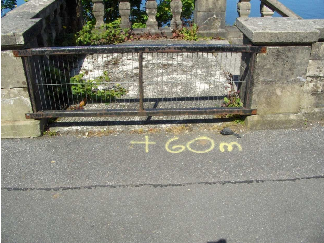
South wall, Chainage 60: Stairway closed
